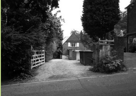
Extensions out of keeping with attractive architecture of historic building
